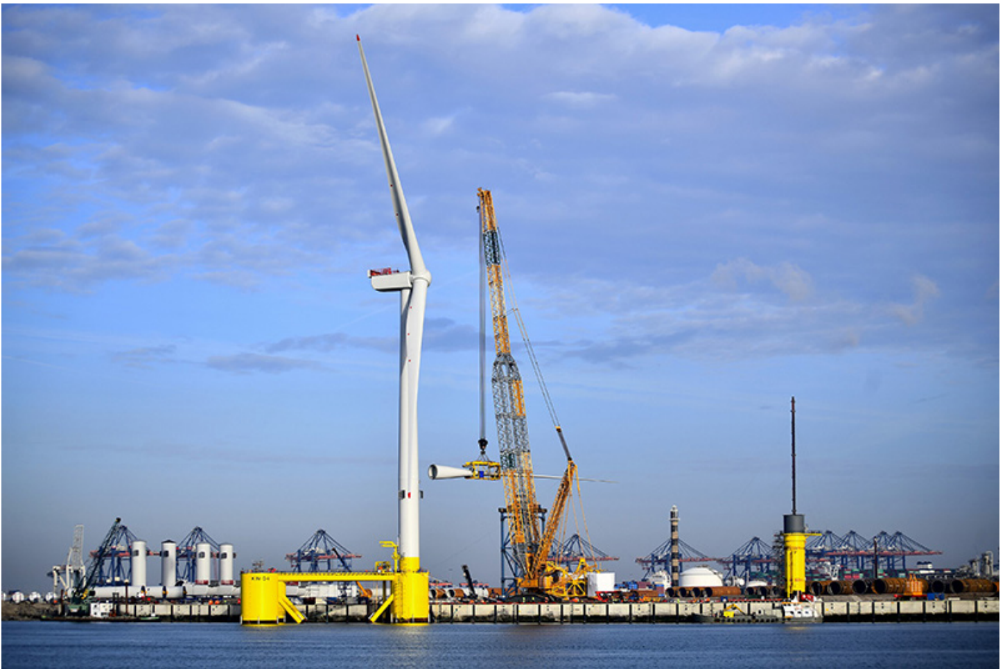
9.5 MW floating wind turbine for Scotland's Kincardine Offshore Wind project at assembly dock in The Netherlands. Photo courtesy of Principle Power
