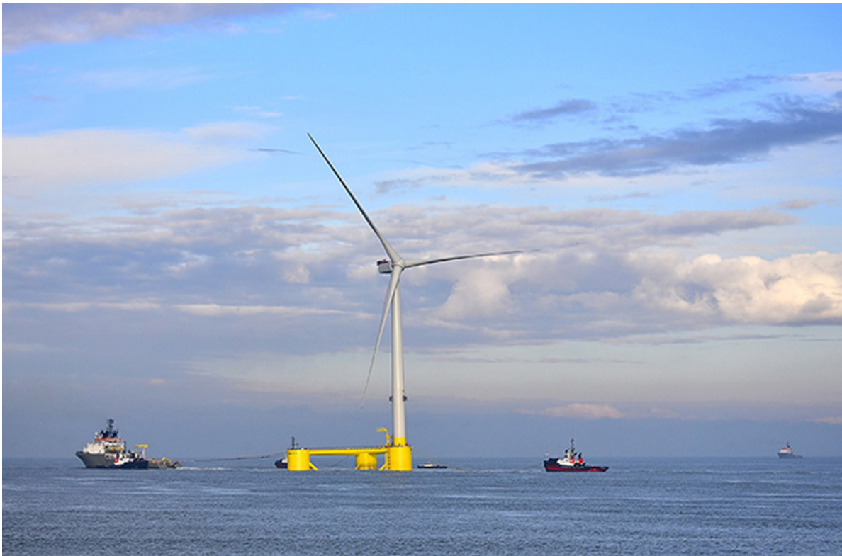
9.5 MW floating wind turbine being towed to Kincardine Offshore Wind project off coast of Aberdeen, Scotland. Photo courtesy of Principle Power
