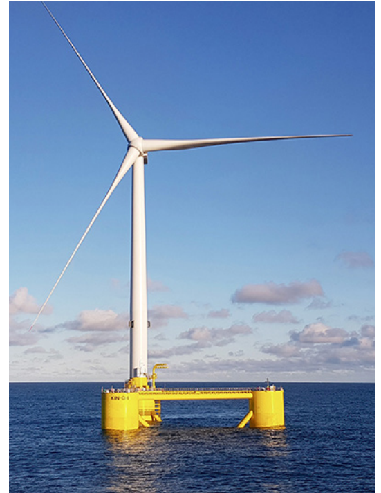
9.5 MW floating wind turbine deployed at Kincardine Offshore Wind project off coast of Aberdeen, Scotland. Photo courtesy of Principle Power
